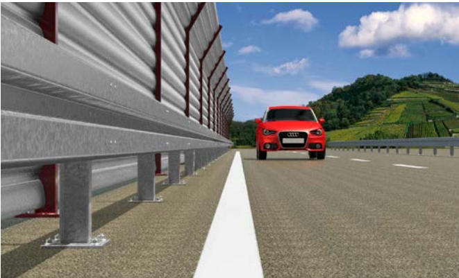
Noise protection walls
