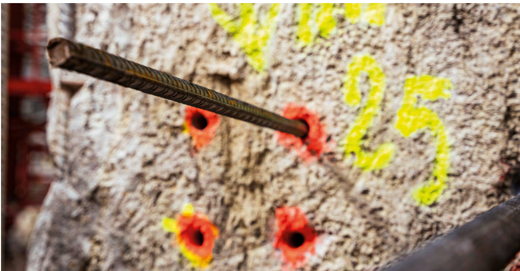
A post-installed rebar on a construction site.
