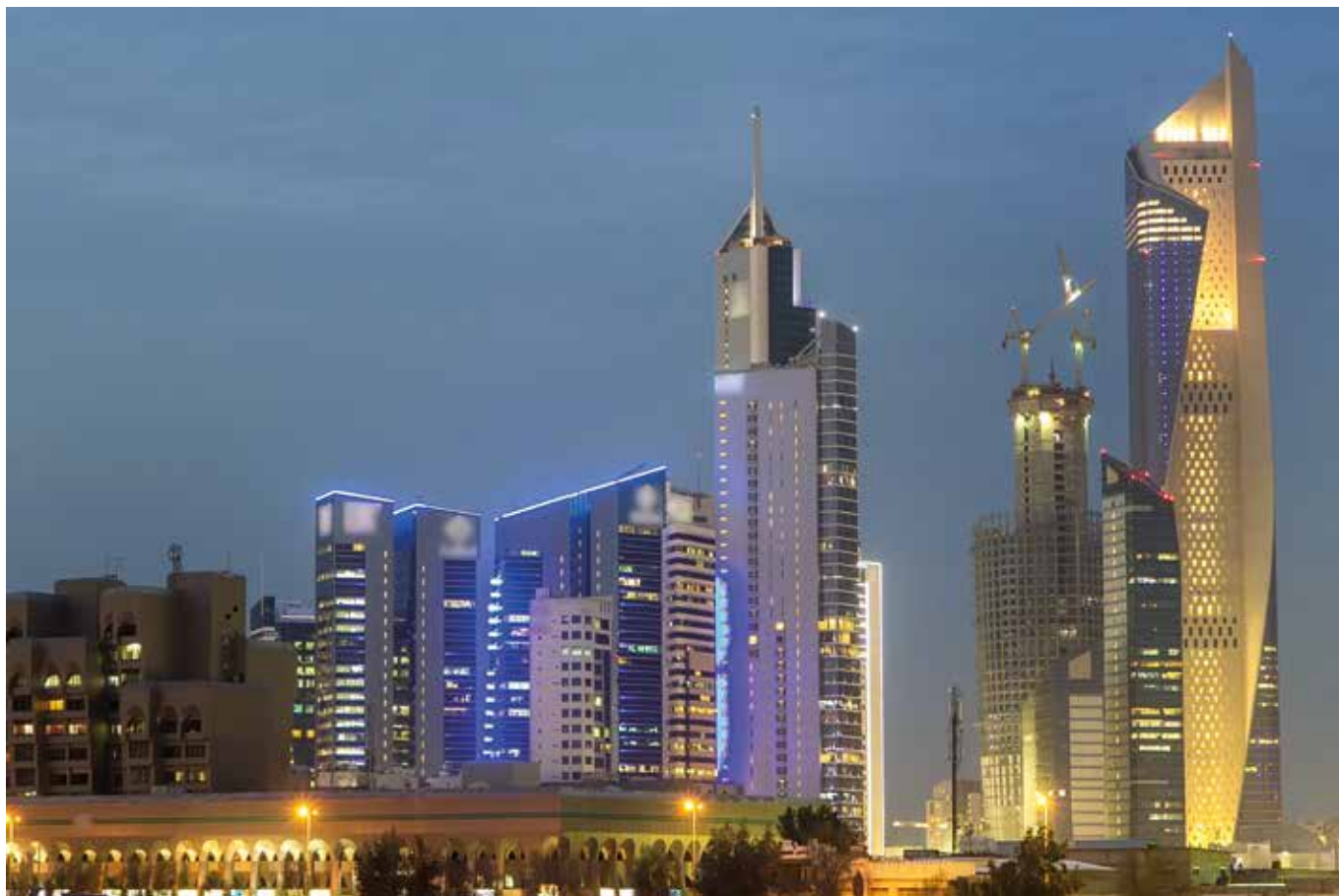
Al Hamra Tower · Kuwait
